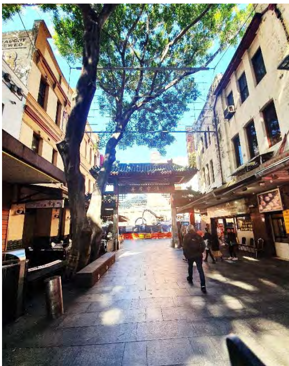
Figure 4.62 Internal (secondary) view from the shared zone between the gates, facing south featuring north elevation of the south gate.
